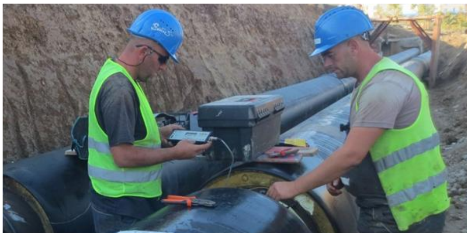
Fig. 7.1 Images from the works on network rehabilitation
