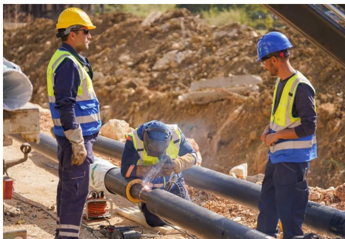
Fig . 7. 1 View from the works on the network expansion and rehabilitation of heating networks
