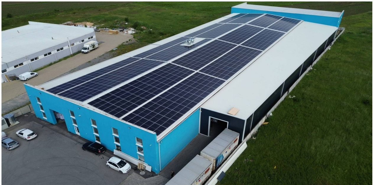
Fig . 3. 2 View from the realization of a generator for self-consumption, legal entity 100 kW
