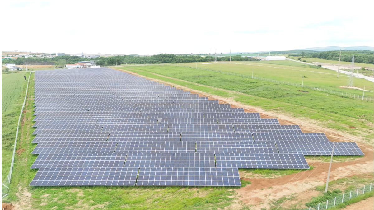
Fig . 3. 1 View from the realization of a solar generator - ELEKTROHETA LLC. Capacity 3000 kW, Ferizaj
